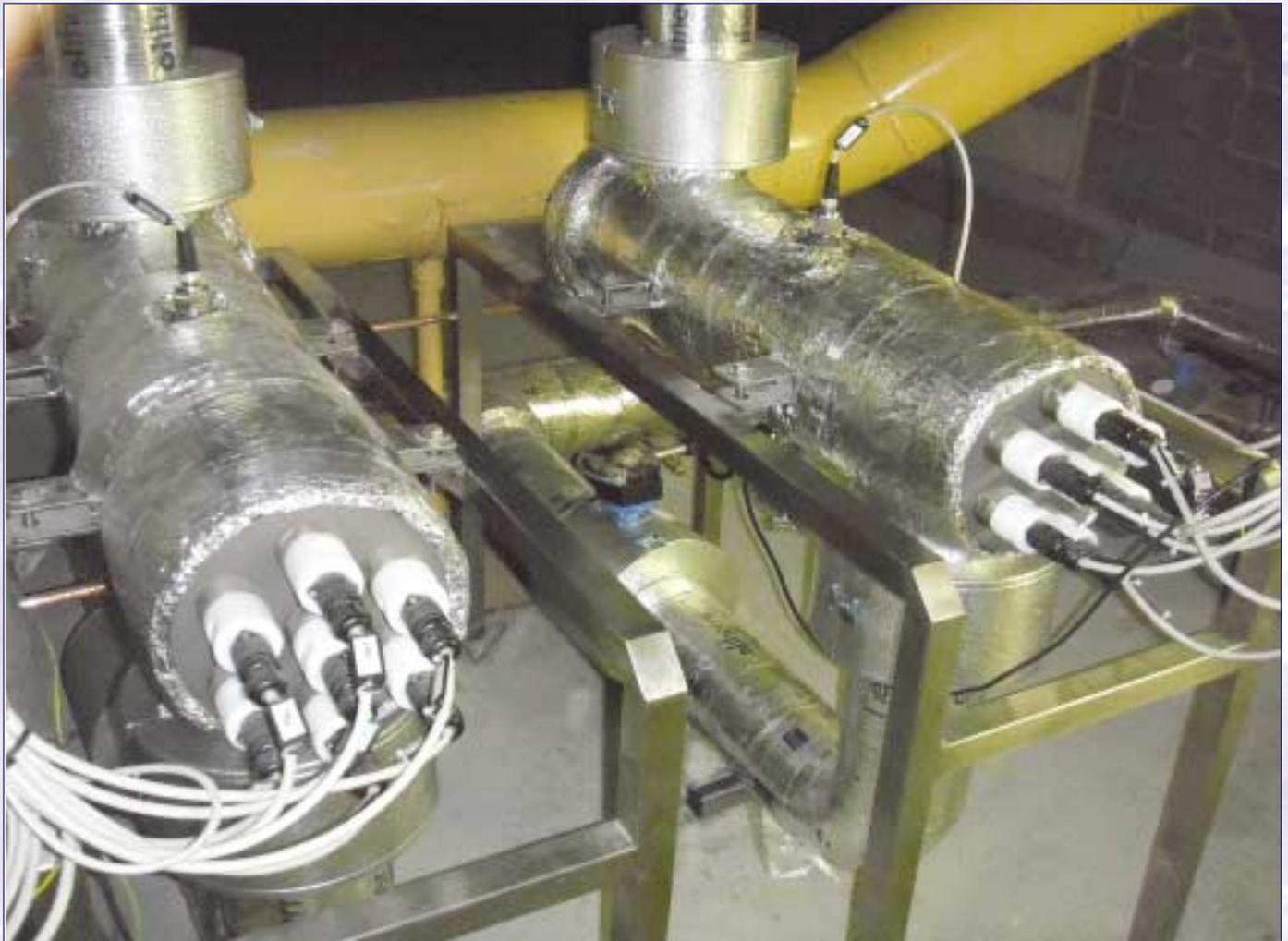
*Skanska were keen to implement the environmentally friendly Titanium AOP system at the Royal London Hospital where innovation and utilising new ideas are part of the hospitals core values. The two AOP 50 units shown have been installed in parallel to provide the level of treatment required by Skanska in a demanding and prestigious hospital environment.*
