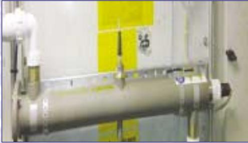
◀ AOP5 fitted to a cooling tower at Kent County Council removing the need for biocide chemicals.
