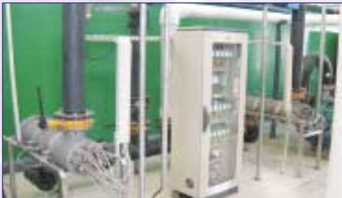
◀ Two AOP100's treating process water at an electronics manufacturer in China.
